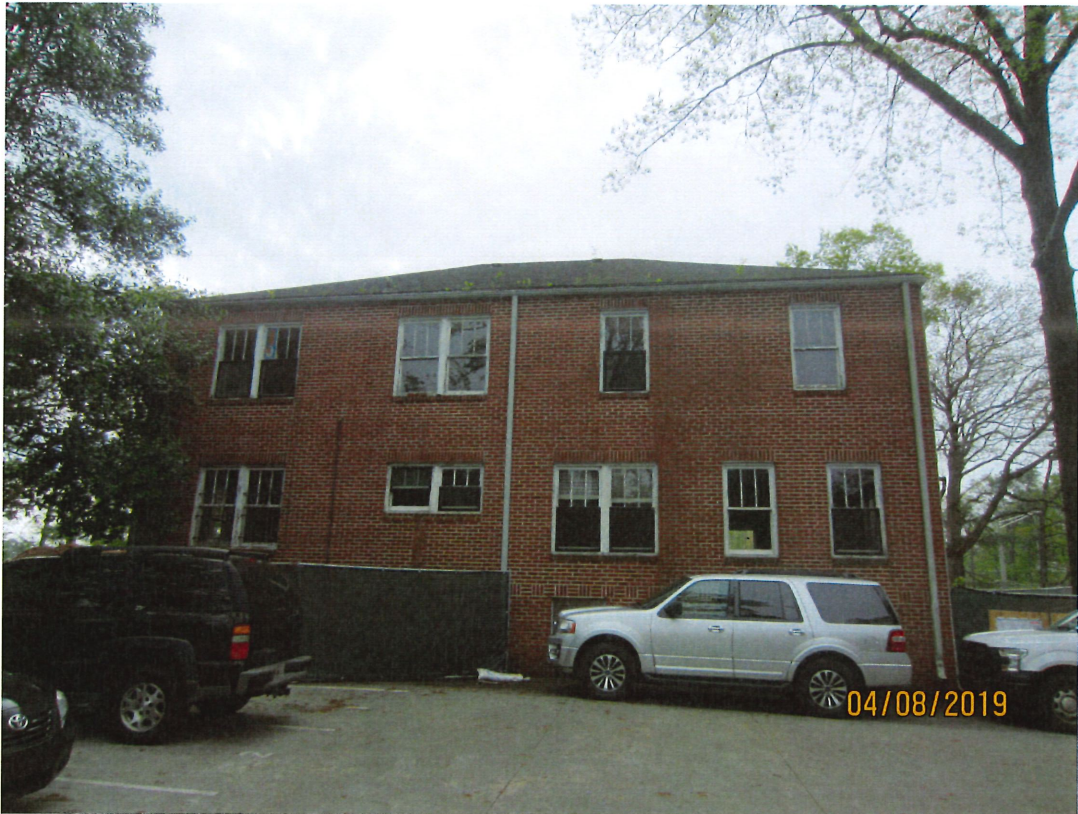
Photograph 3: Resource 1 west elevation, looking southeast.
