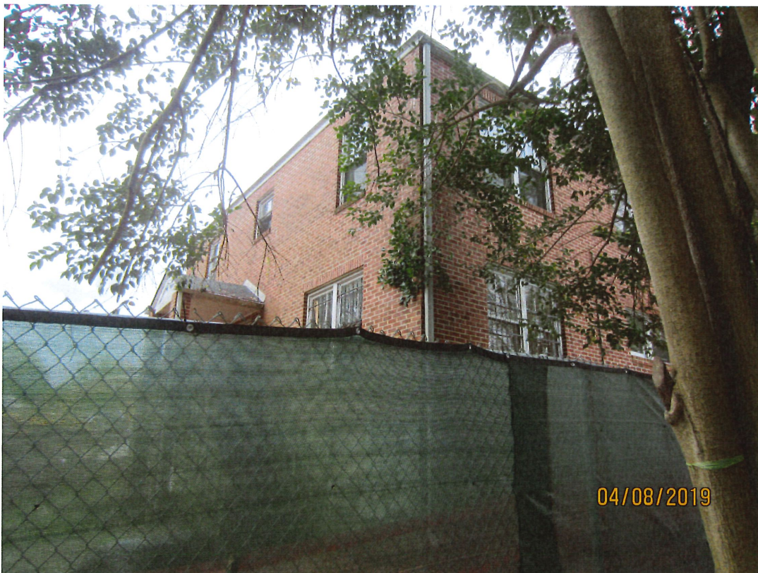
Photograph 4: Resource 1 oblique showing rear (north) and west elevations, looking south.
