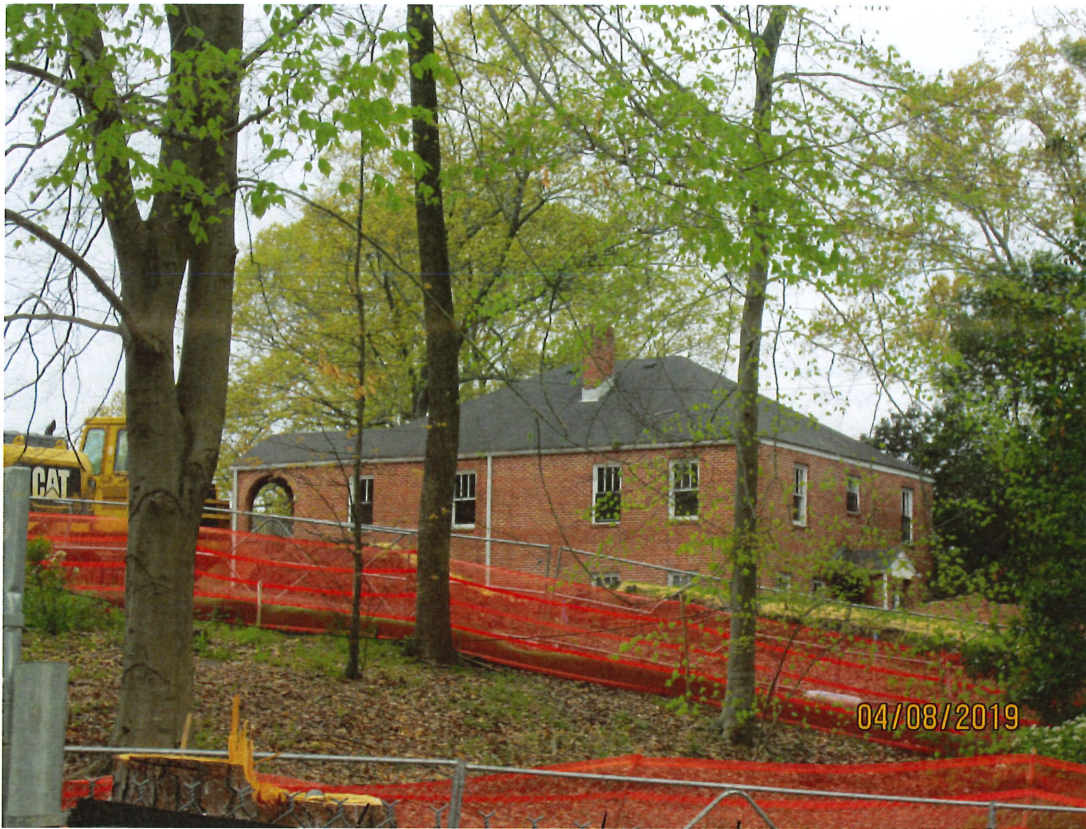
Photograph 5: Resource 1 oblique showing east (side) and rear elevations, looking west.
